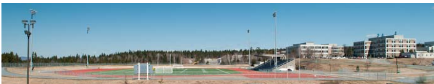
Renovated Canada Games Stadium at Tucker Park 2011
